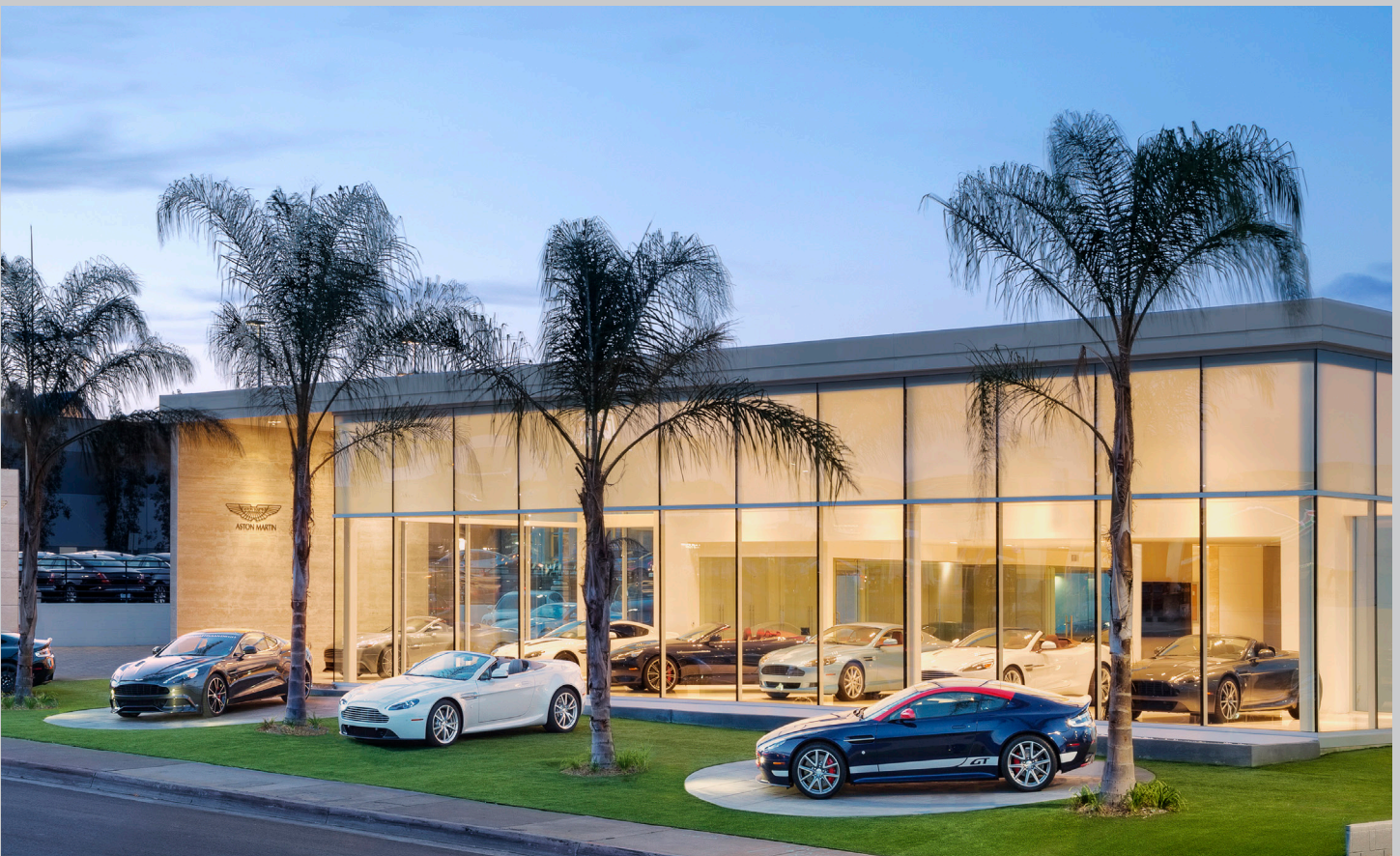
Curtainwall with Low-E Glass IG Units
